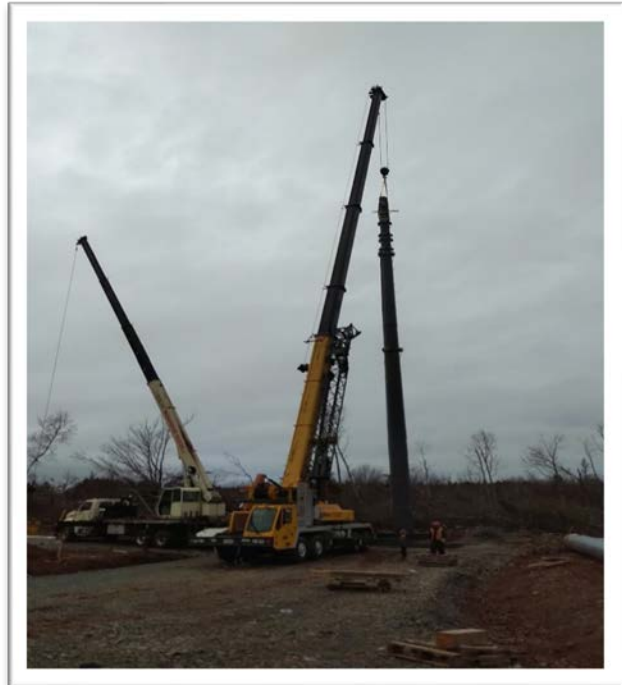
Work on the River John Tower progresses in 2023.
