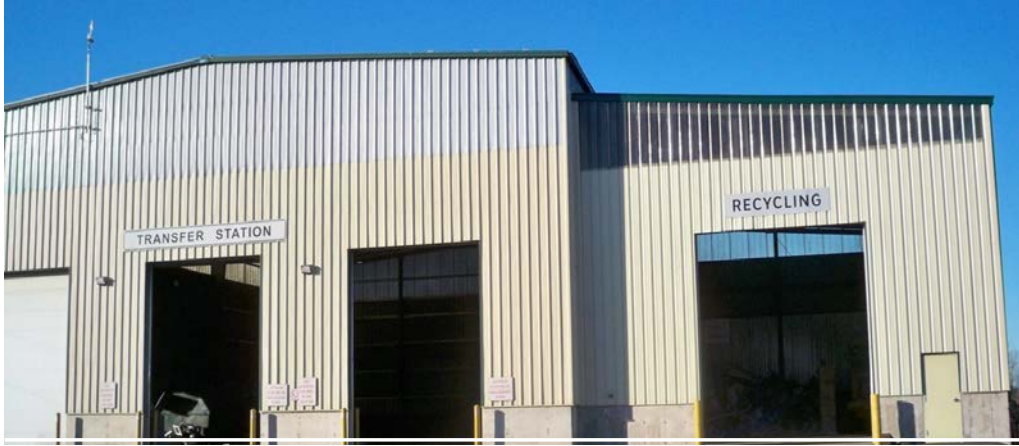
Transfer Station & Recycling Building
